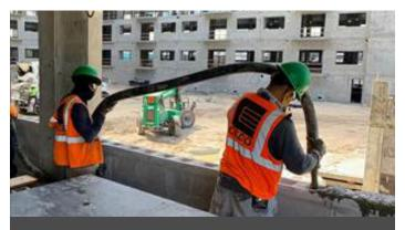
To provide perimeter protection against hurricanes, masonry blocks are set, reinforced and those cells are grouted full of concrete.
