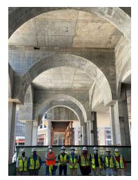
Ceco Concrete provided full concrete framing services for the development's hotel and office buildings that site atop a parking ramp, placing concrete for all foundations, columns, walls and arches as well as elevated reinforced-concrete and post-tensioned concrete decks.
