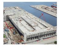
The beam-and-slab garage has five levels, totaling 1 million square feet of contact area, with 60-foot-long spans. The long spans led structural engineer Ammann & Whitney to design a concrete structural system for PT beams and decks. Ceco used steel beam and table formwork systems to construct the 20-foot
