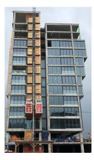
Ceco provided structural design and turnkey frame services (excluding foundations), taking the project from conceptual drawings to a complete designbuild package. A one-way posttensioned (PT) flat plate system was selected to reduce clear story heights and create a flat ceiling for the apartments. Other structural elements include a C-shaped stairway, one elevator core and two straight shear walls.
