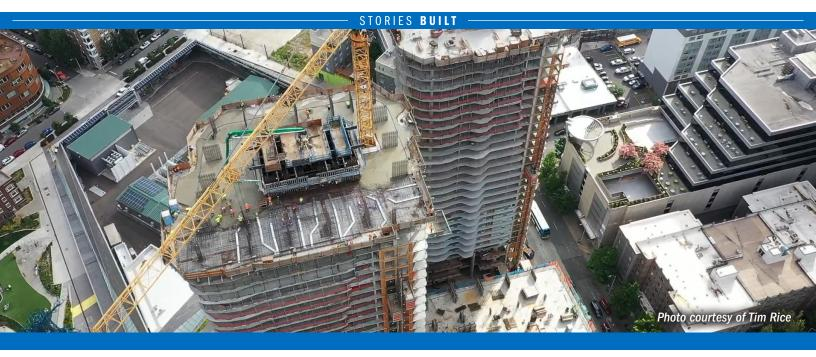
Ceco Concrete is providing full concrete frame services—including all formwork, concrete supply, shotcrete and pump, place and finishing work—for two 48-story residential towers over five below grade parking levels in the heart of Seattle's Denny Triangle Urban Center Village. The project also includes an 8-story podium structure that will house a state-of-the-art concert venue that the structure was modified to include after construction had started.
