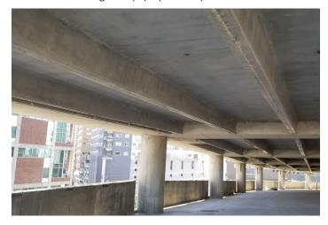
Construction began December 2019. Ceco provided the concrete frame with our client Balfour Beatty providing the materials, which included pumping, placing and finishing all concrete for the 650,000-sq-ft building. The Link's structural system is wide-module, one-way concrete pan construction, which enabled the greater spans
